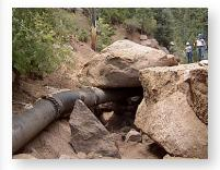
80% of our community's potable water supply during times of high demands. While Utilities' primary Northfield infrastructure was not damaged, a critical secondary component, the Pine Valley Pipeline, was exposed and undermined by storm and debris flows, causing damage estimated to be near \$6 million. Of course, to make these repairs Utilities must take steps to protect its infrastructure from future flood flows.
