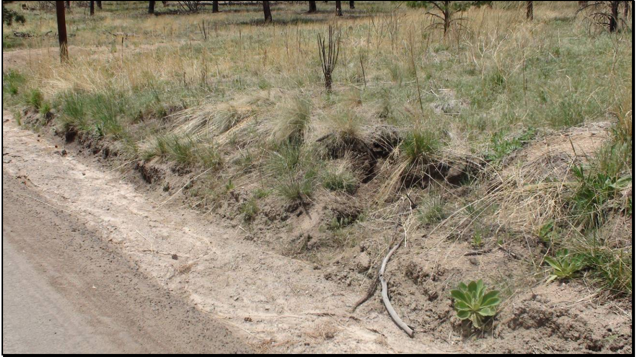
Figure 17. Sediment transported down the ditch line of a road in the Trail Creek Watershed.
