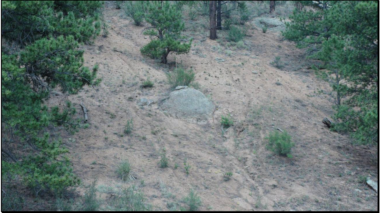
Figure 15. Surface erosion indicating rill erosion above road cut.
