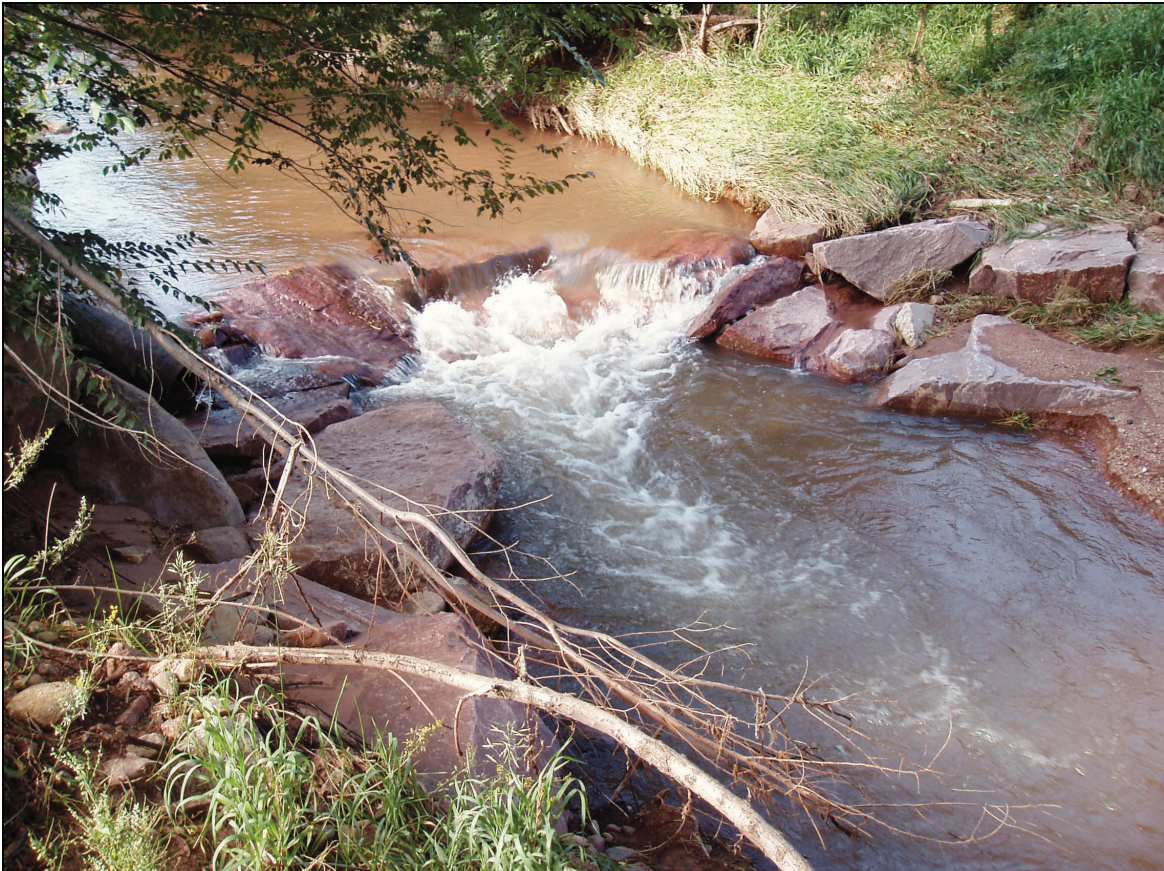
Cross Vane Structure on Fountain Creek below 21 st Street Bridge, El Paso County, CO.
