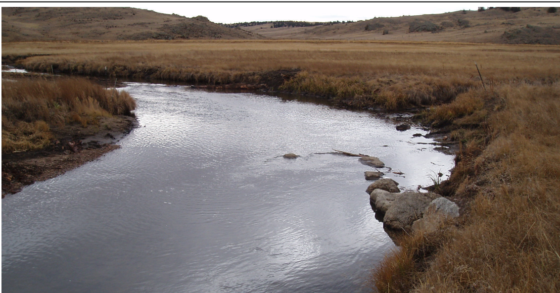
Example of a boulder J-Hook Vane. Tarryall River – Eagle Rock Ranch, Park County, CO
