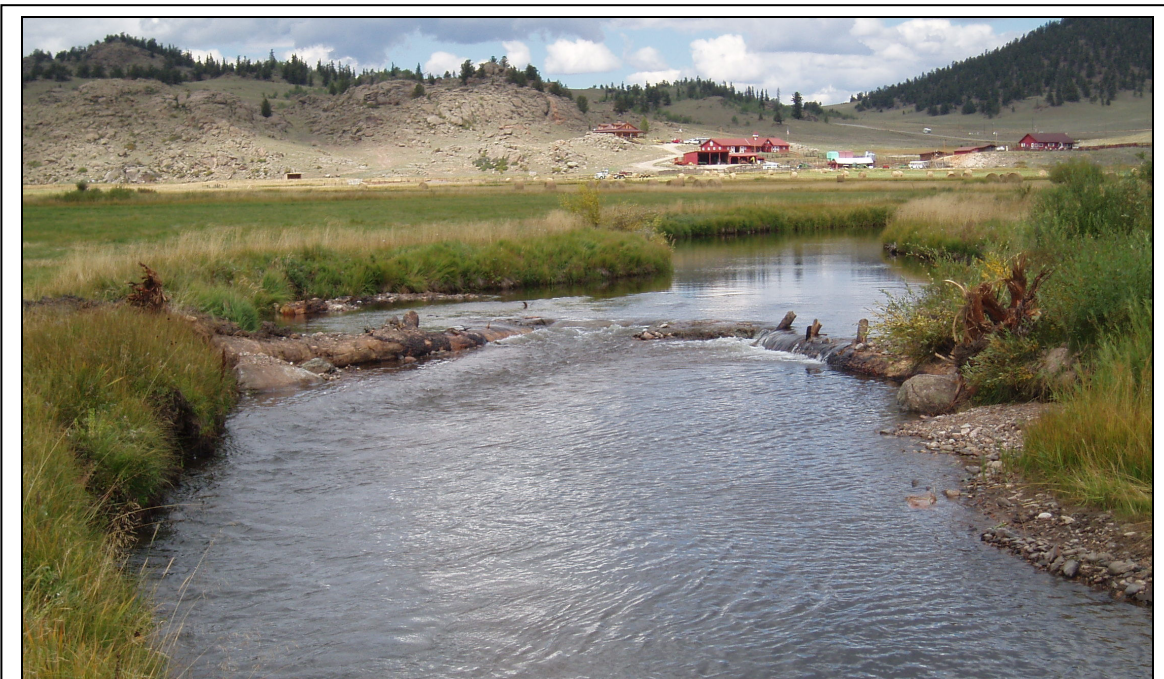
Double Log /Boulder Cross-vane Structure - Eagle Rock Ranch, Tarryall River, Park Co., CO
