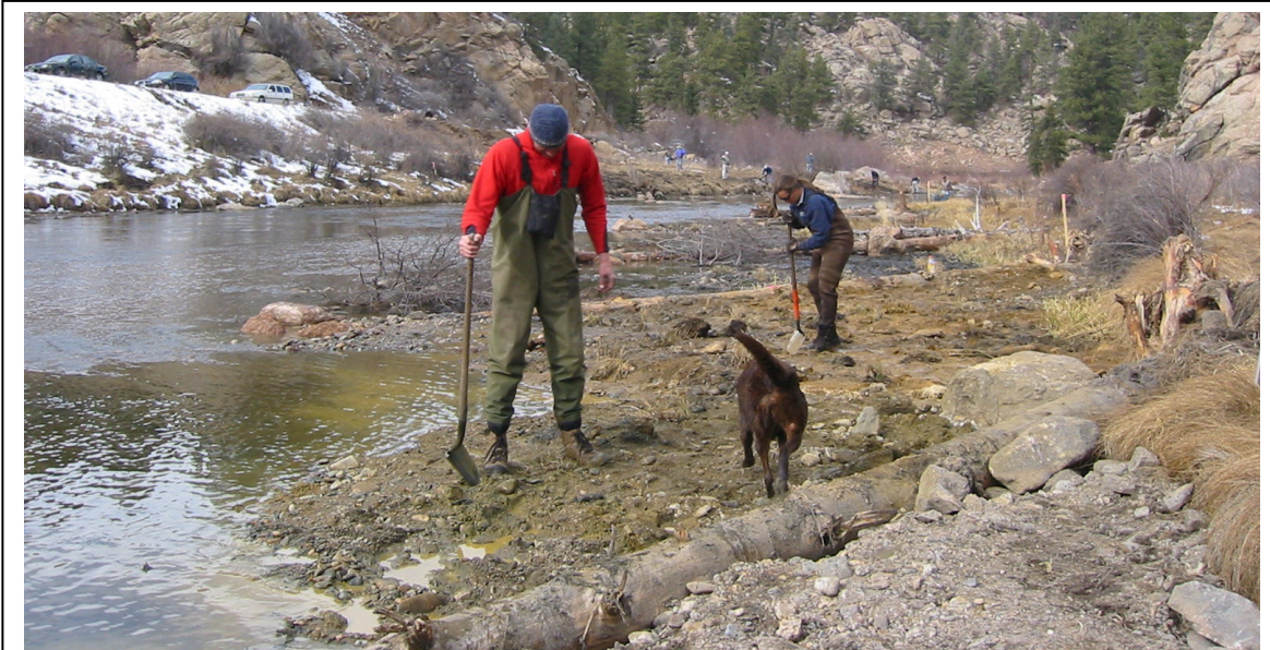
Large wood installed low in the channel to reduce width/depth ratio - South Platte River, Elevenmile Canyon, IFIM Springer Gulch Middle Station. 2004 "Trees for Trout" Demonstration Project
