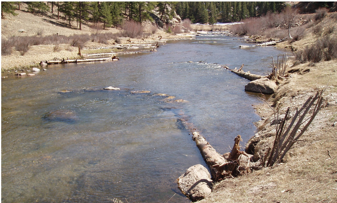
Large wood / boulder J-Hook Vanes - South Platte River, Elevenmile Canyon, IFIM Springer Gulch Middle Station. 2004 "Trees for Trout" Demonstration Project.
