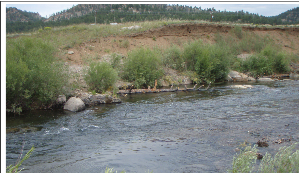
Example of bank full bench structures and a habitat tree along the outside of a meander bend.
