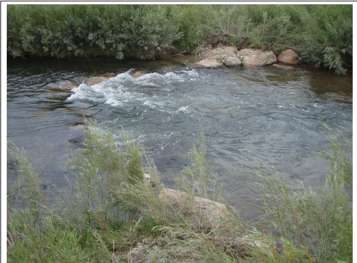
Full Channel Boulder Cross-vane. South Platte River at Lake George, CO.
