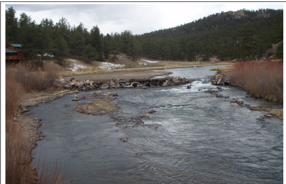
The diversion structure at the upstream boundary of Reach 21 on the S. Platte River in Sportsman's Paradise.
